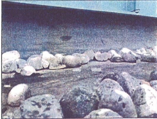
Flashing membrane terminates behind panels on RA 18
