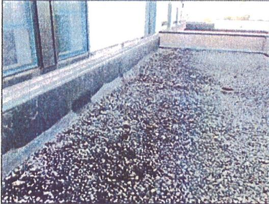
Membrane shrinkage on RA 7
