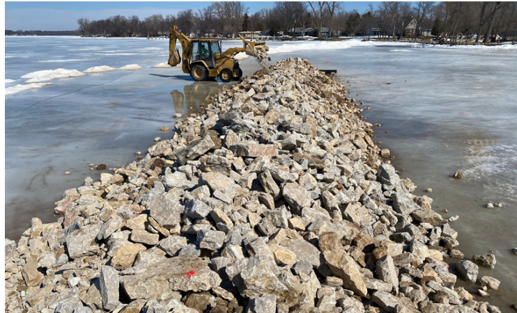
Breakwall Constructed on the Ice
