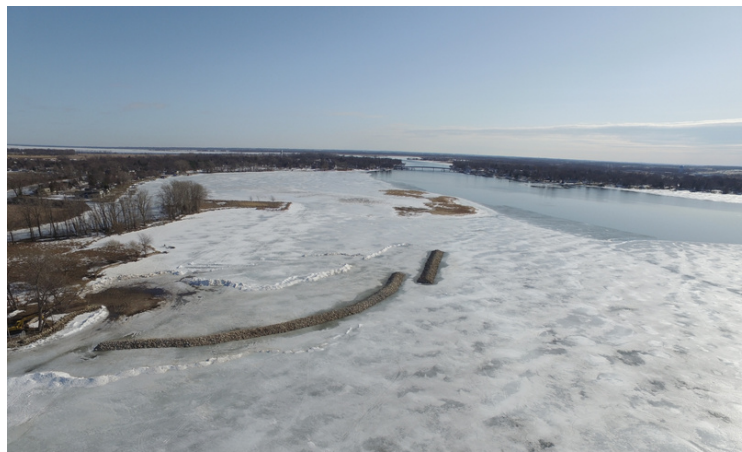
Final Constructed Breakwall on the Ice
