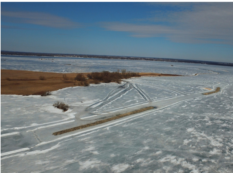
1,000 Feet of Breakwall Installed on the Ice
