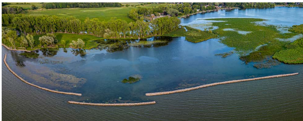
Breakwall project on Lake Winneconne. This 2023 photo shows increased vegetation growth and protection from erosion. Photo Credit: Tim McEnroe.
