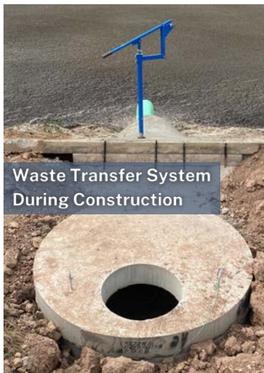
WASCOB During Construction: Inlet Structure (Water And Sediment Control Basin)
