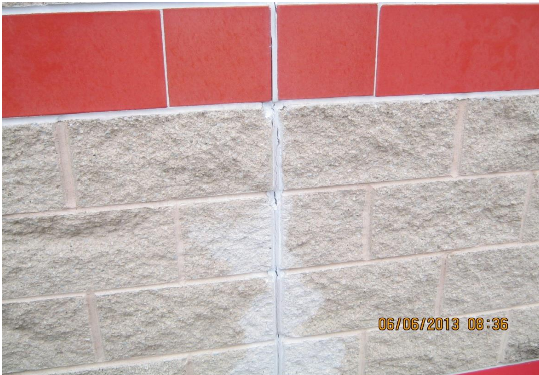
Highway Shop failed mortar joints
