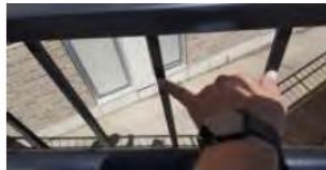
Illustration #5: Left – Shows accessible ramp cutting off access to area well and lower level windows. Right shows a gap larger than 4 inches on center for vertical rails on guardrail.
