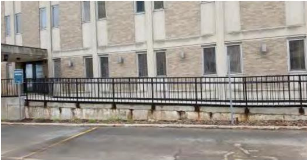
Illustration #4: Existing accessible ramp, indicates concrete deterioration and guardrail rusting
