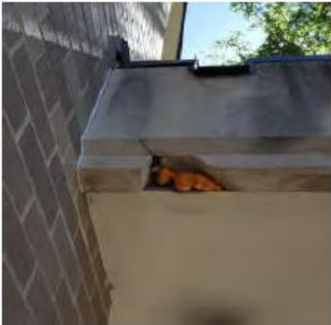
Illustration #7: All – Discoloration indicates water residue from drip edge above. All- indicates panel failure from steel pin holding the panel in place.
