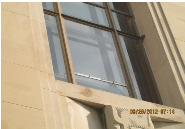
Deteriorated window framing replaced
