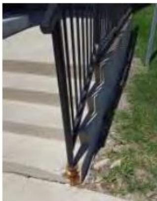
Illustration #6: Left – Missing concrete corner and interstitial moisture. Right-Streaking indicates embeds for railing too close to the surface of concrete
