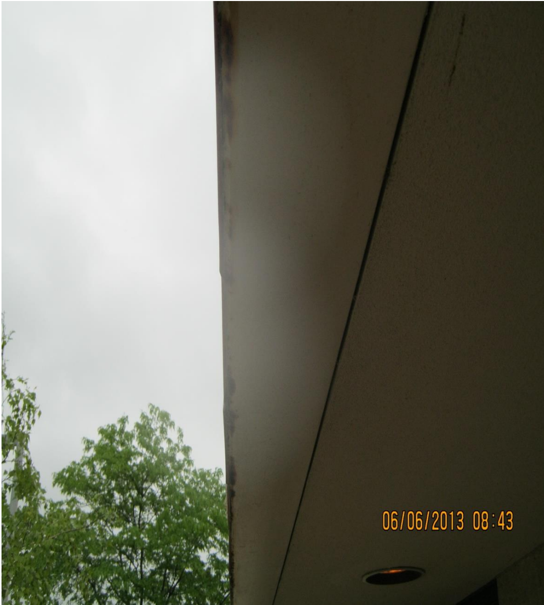
Highway Shop water damaged façade
