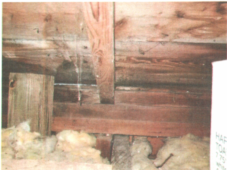
Photo taken in LOFT of rough-sawn Full-dimension 2x4's + plank roofing 4x4's
